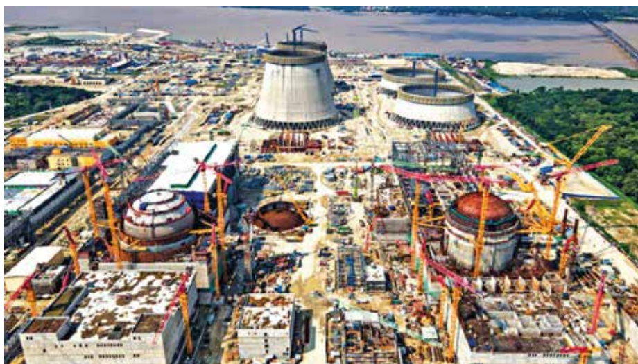
Rooppur nuclear power plant
