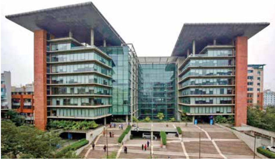
Grameenphone Head Office at Bashundhara Residential Area
